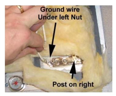
Screw the tall hex nuts onto each side. The left hex nut should be pressing the ground wire ring terminal down on top of the thermostat tab. Tighten both tall hex nuts snug. (Do not overtighten)
